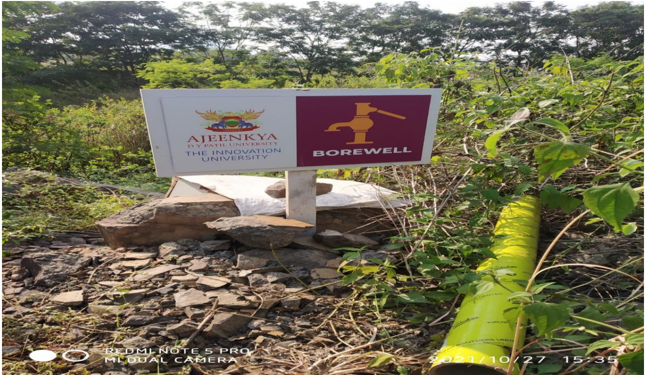
Bore well is provided in the campus in the vicinity of lake
