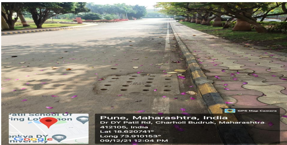
Road Cross Drainage Work which was connected to the chambers located in the campus
