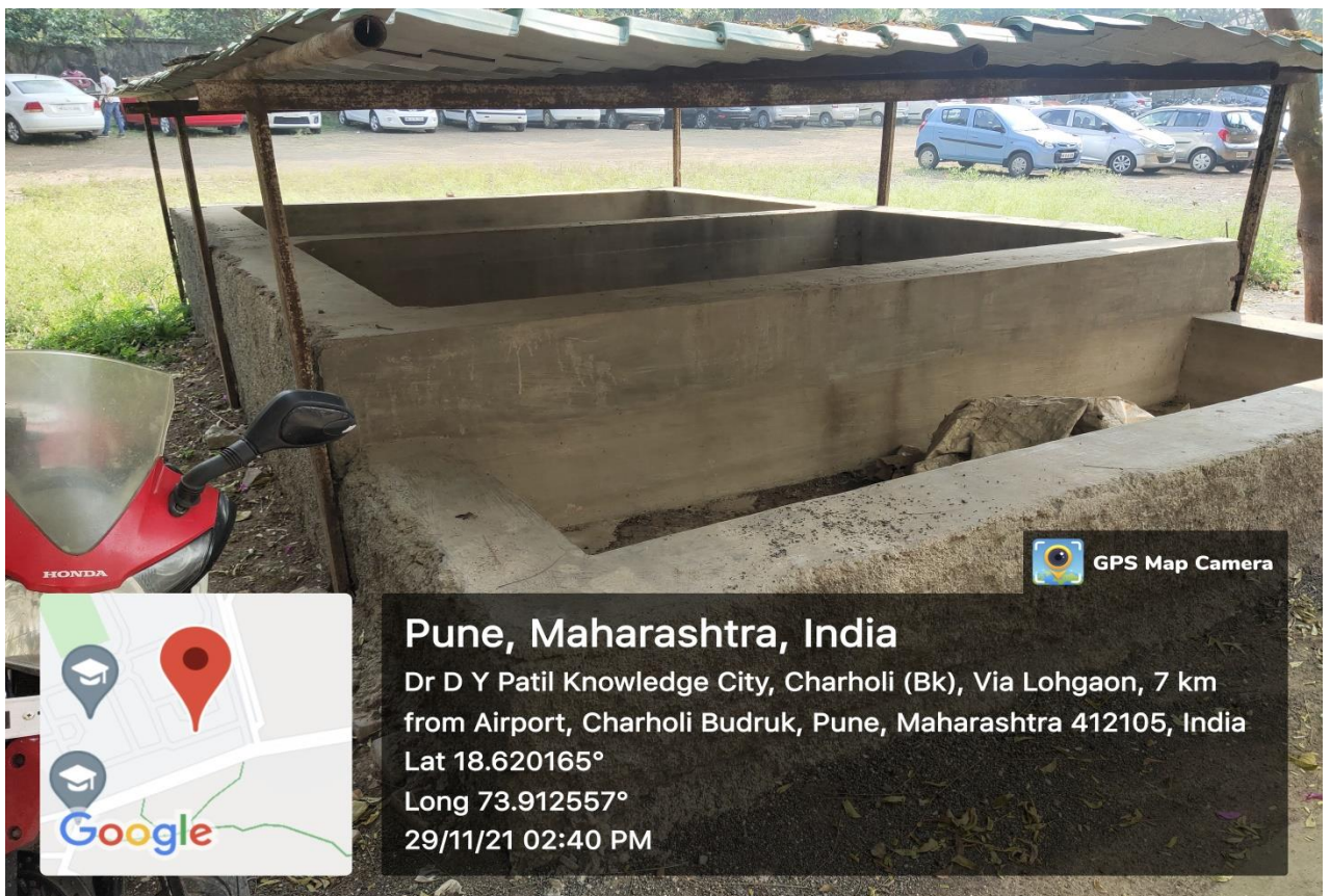
Ground Water Storage Tanks are Located at different locations in the Campus
