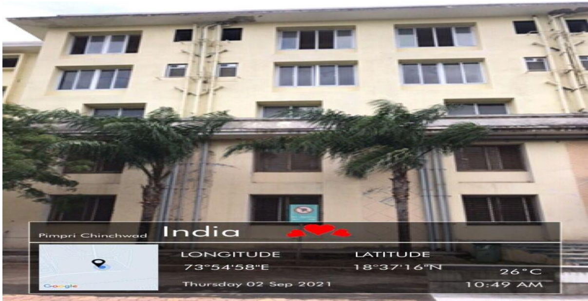
Roof water pipes are connected to chambers
