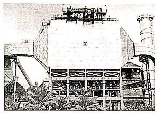
At the sugar factory, we observed the equipment responsible for air pollution control i.e Electrostatic precipitator. The model present at the factory was of Thermax APC Business.
