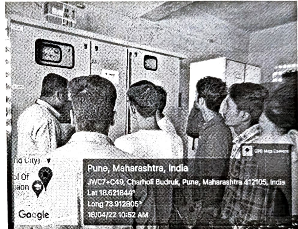
Decoding the monitoring system
